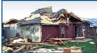
**F2 Considerable:** Roof structures are damaged, mobile homes are destroyed, debris becomes airborne (**missiles** are generated), large trees are snapped or uprooted.
