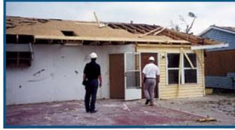
**F1 Moderate:** Roof surfaces are peeled off, windows are broken, some tree trunks are snapped, unanchored mobile homes are overturned, attached garages may be destroyed.
