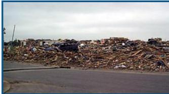
**F5 Incredible:** Strong frame houses are lifted from foundations, reinforced concrete structures are damaged, automobile-sized missiles become airborne, trees are completely debarked.
