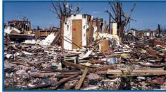
**F4 Devastating:** Well-constructed houses are destroyed, some structures are lifted from foundations and blown some distance, cars are blown some distance, large debris becomes airborne.
