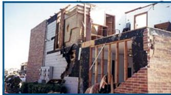
**F3 Severe:** Roofs and some walls are torn from structures, some small buildings are destroyed, non-reinforced masonry buildings are destroyed, most trees in forest are uprooted.
