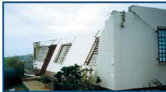
**C4 Extreme:** Extensive damage is done to roofs, windows, and doors; roof systems on small buildings completely fail; some curtain walls fail.
